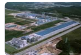
Daejeon Gymsum Plant
